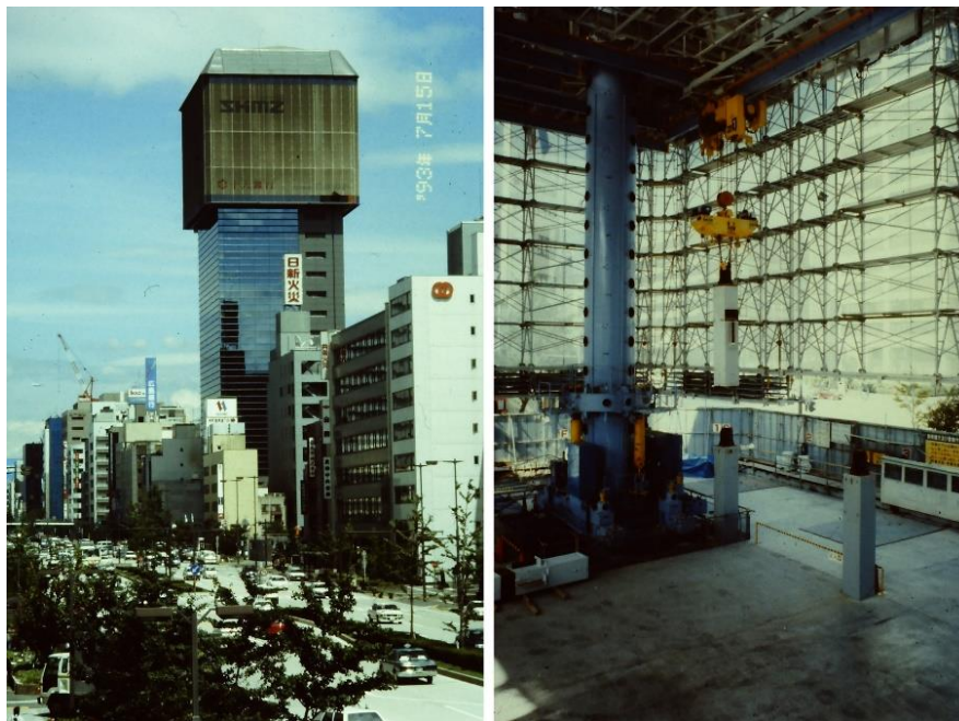
Figure 6 The pioneering automated construction site “SMART” developed by Shimizu Corporation (photo: T. Bock)
