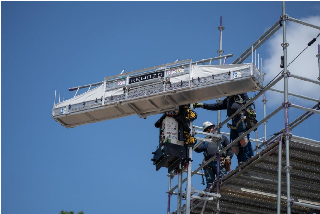
Figure 19 KEWAZO's LIFTBOT in operation on a construction site (photo: KEWAZO GmbH)
