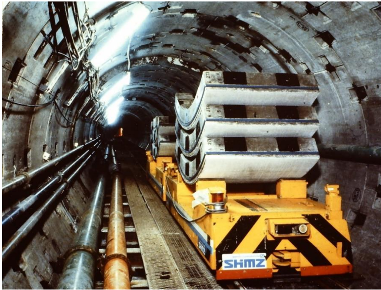
Figure 5 Teleoperated construction robot for tunnel construction (photo: T. Bock)
