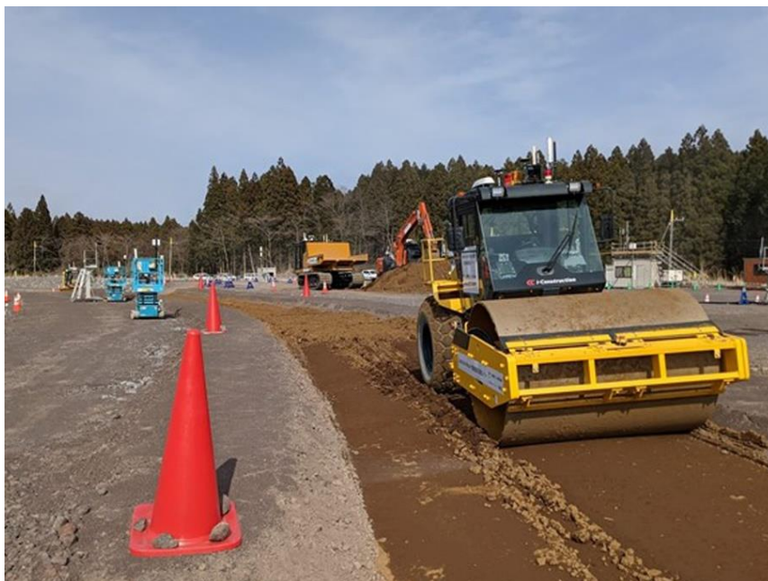
Figure 6 Autonomous heavy machinery fleet for infrastructure projects (Photo: T. Bock)
