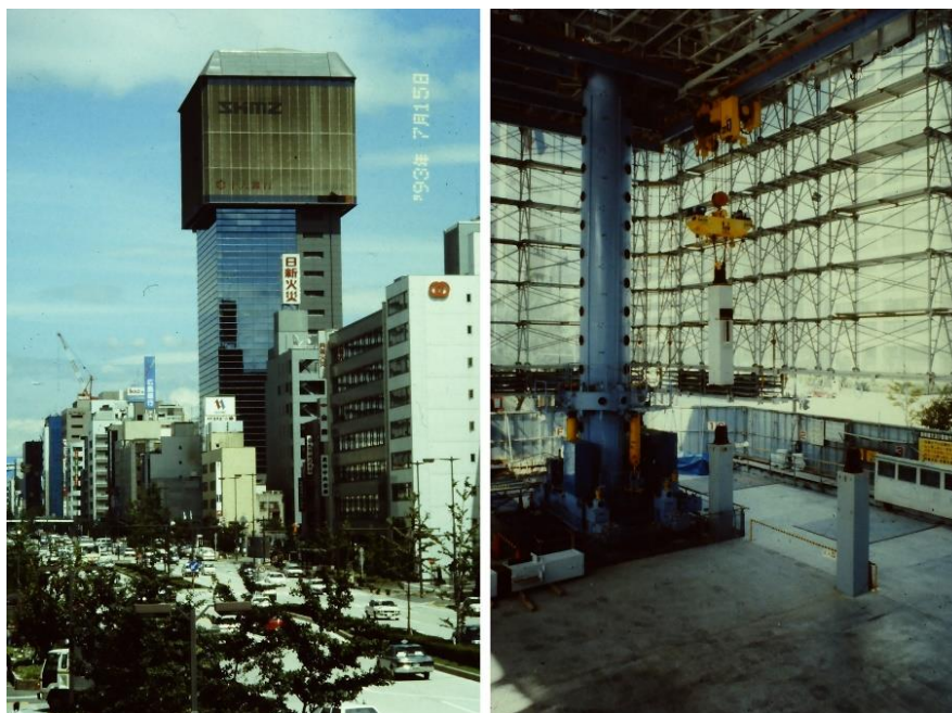
Figure 4 The pioneering automated construction site “SMART” developed by Shimizu Corporation (photo: T. Bock)
